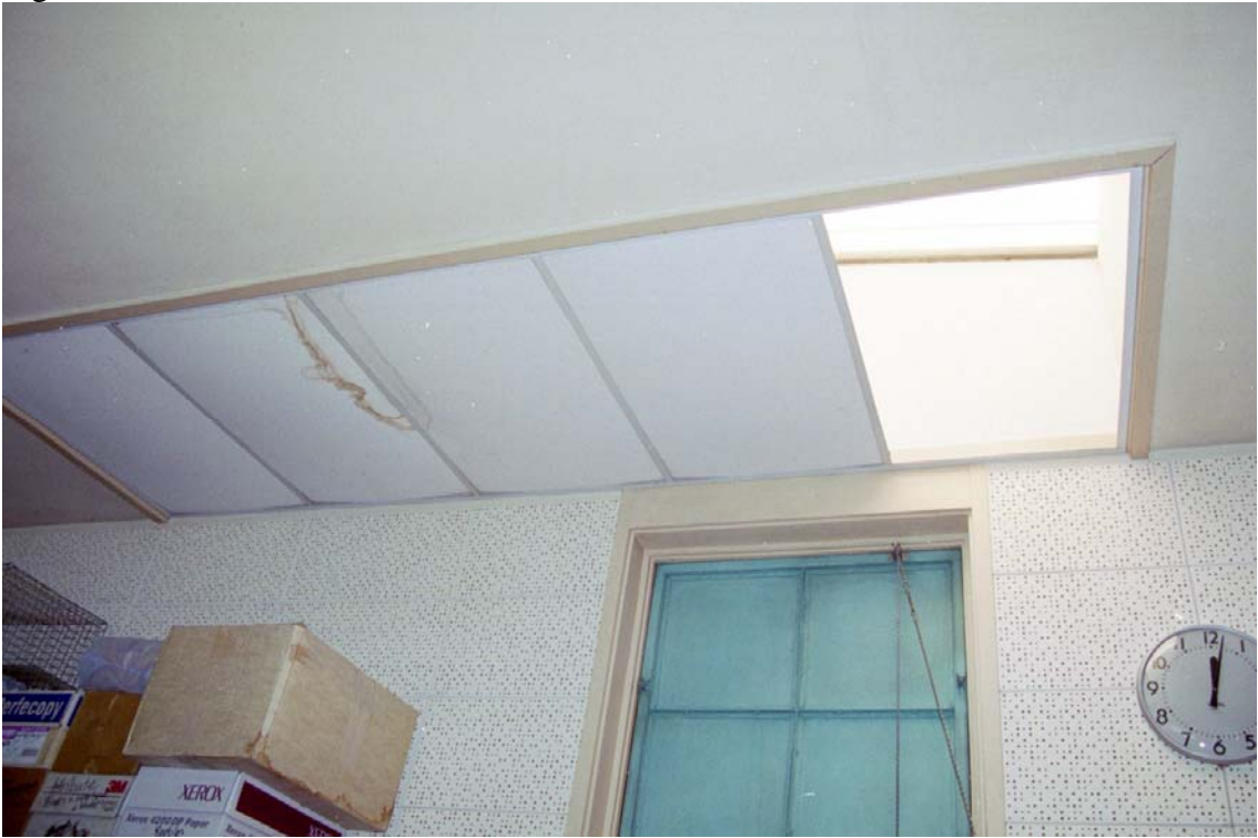
Figure 3: Skylight inside classroom with water leakage
