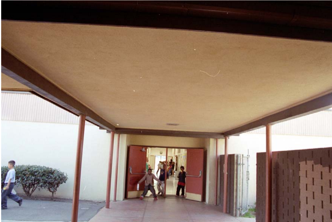
Figure 12: Covered Walkway between units 'B' and 'A' with plaster ceiling
