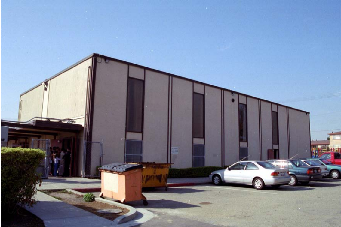
Figure 10: East wall of Multi Purpose Building
