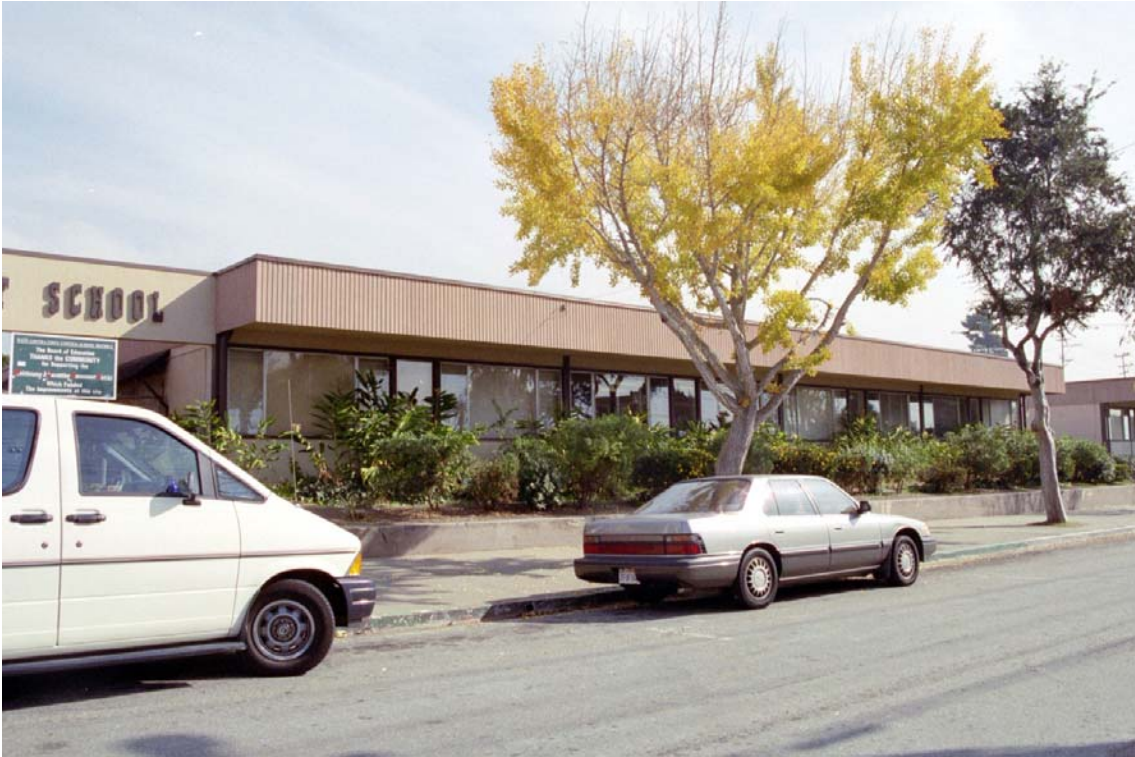
Figure 8: Exterior Longitudinal (west) wall (unit 'B')
