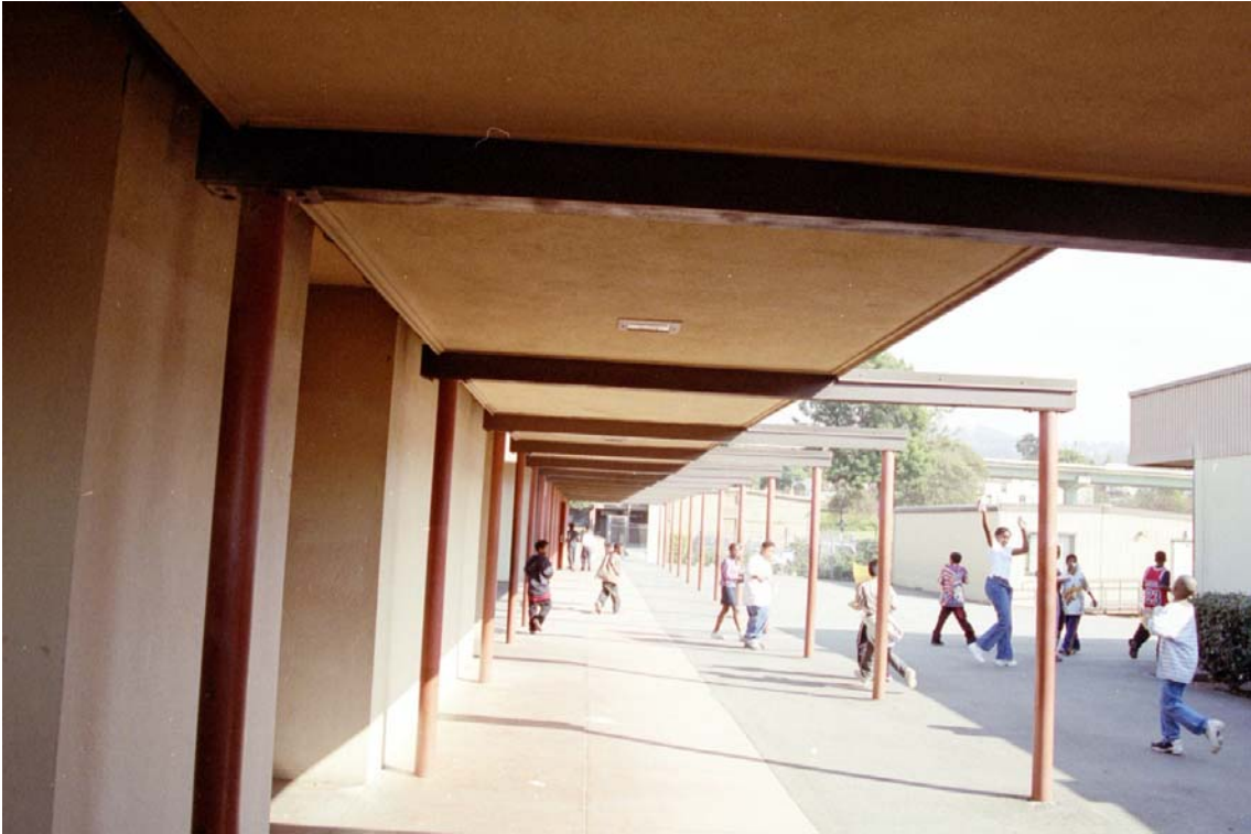
Figure 4: Covered Walkway (Not attached to the classroom building on left)
