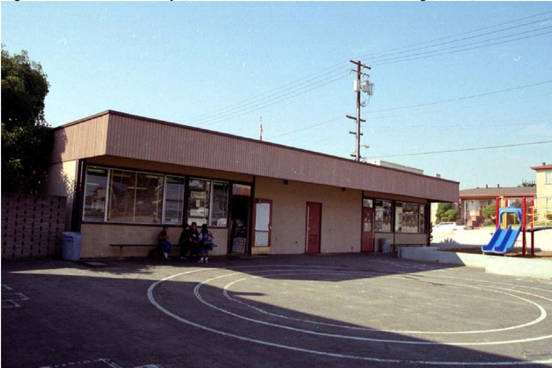
Figure 5: East wall of Kindergarten Building
