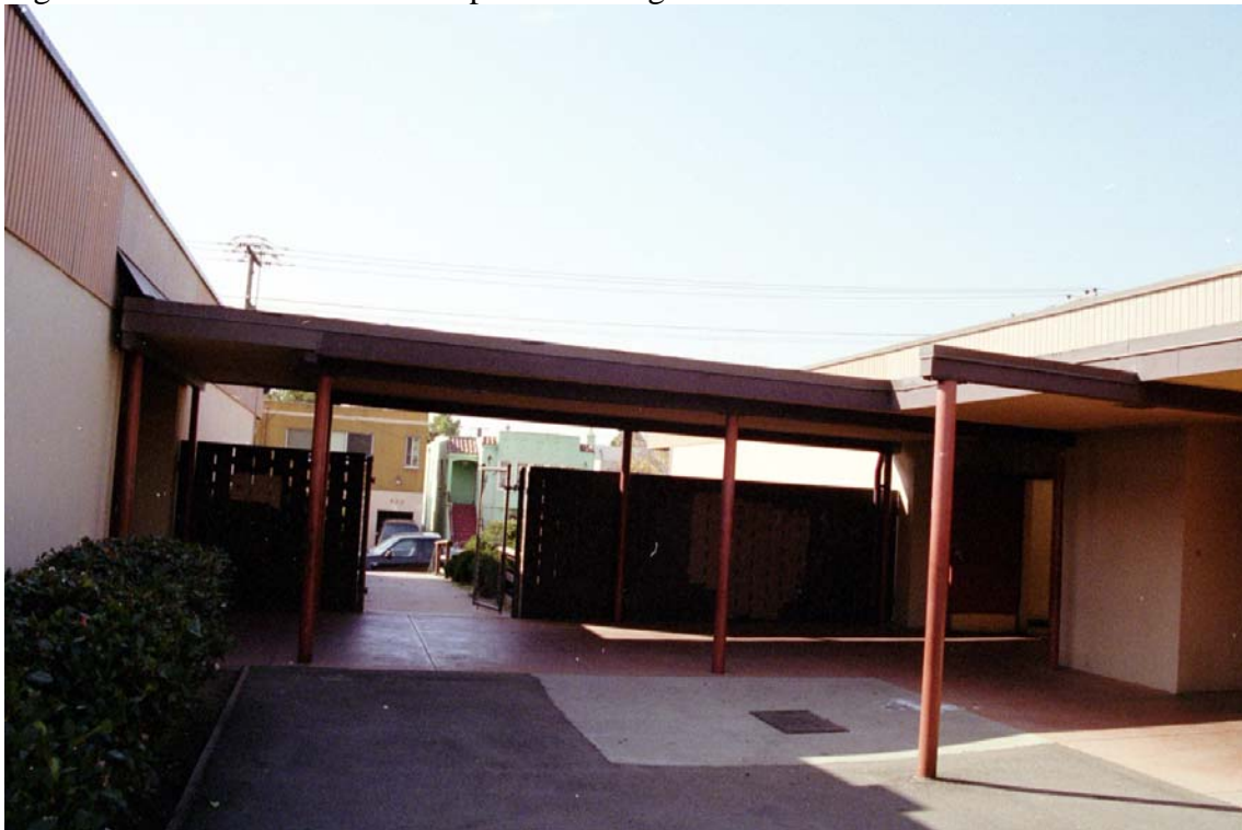
Figure 11: Covered Walkway between units 'B' and 'A' (seismic gap at the left)
