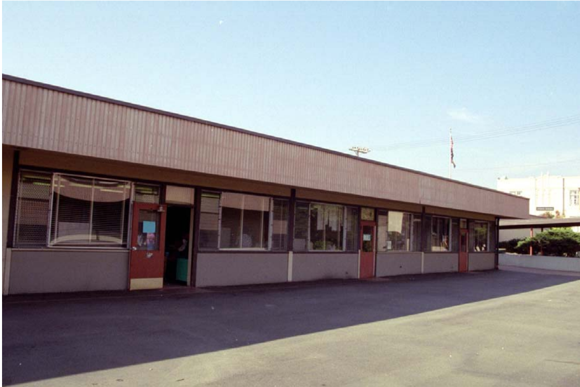
Figure 6: East wall of Classroom building (unit 'B')
