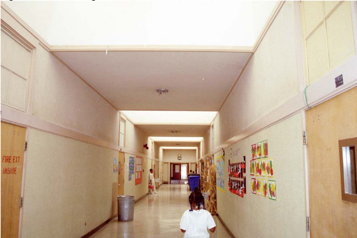
Figure 9: Interior Corridor showing Skylights
